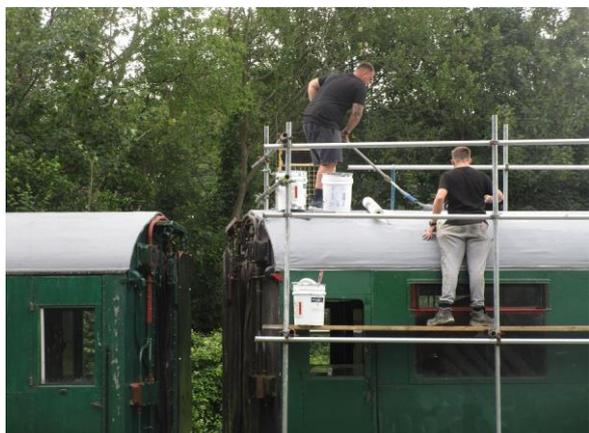
Here we see the contractors installing the new roof to '61. The process involves painting on a layer of primer onto the roof canvas to dry out the roof surface and to provide a layer for the membrane to adhere to. Then layers of liquid membrane get applied and adding a fine flexible mesh with more layers of liquid membrane.
