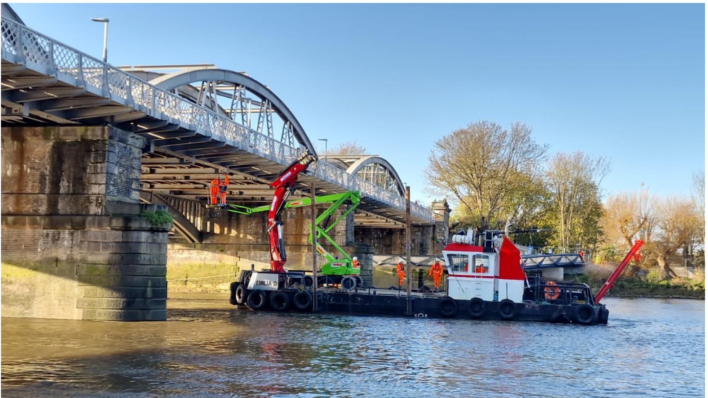
Repairs under way at Barnes Bridge (Network Rail photo)
