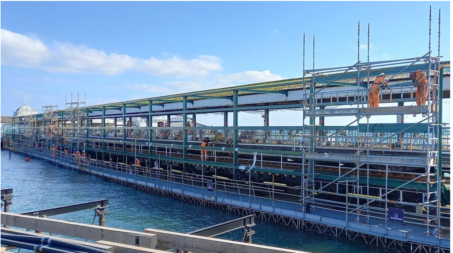
Work under way at Ryde Pier Head station. Photo: Network Rail
